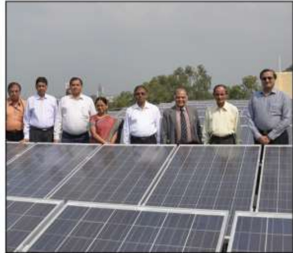
Secretary, Ministry of Coal Govt. of India Sri SK Srivastava, along with Sri AK Debnath, CMD, CMPDI and others with Roof Top Solar Power Plant
