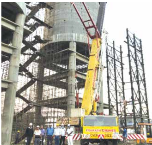
Figure 2 Showing construction of Silo for JVR OC CHP, SCCL.
