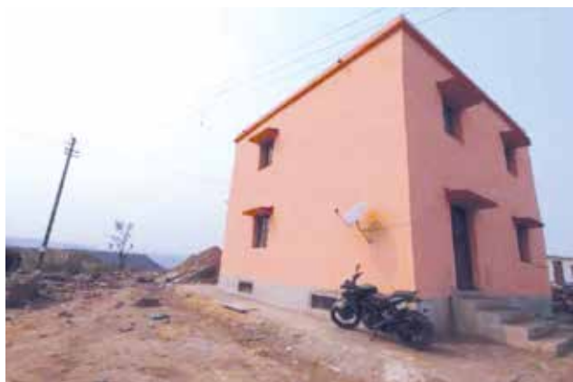
Figure 1 Prototype Building constructed at Jagannath Area, MCL for S&T project titled constructing structures on backfilled opencast coal mining- an attempt to suggest viable methodologies
