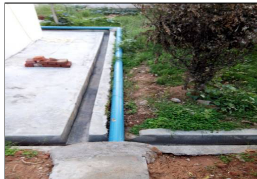
Figure 62: Pipes to collect rain-water from the roof top of the building in CMPDI, RI-VI, Singrauli, Madhya Pradesh.
