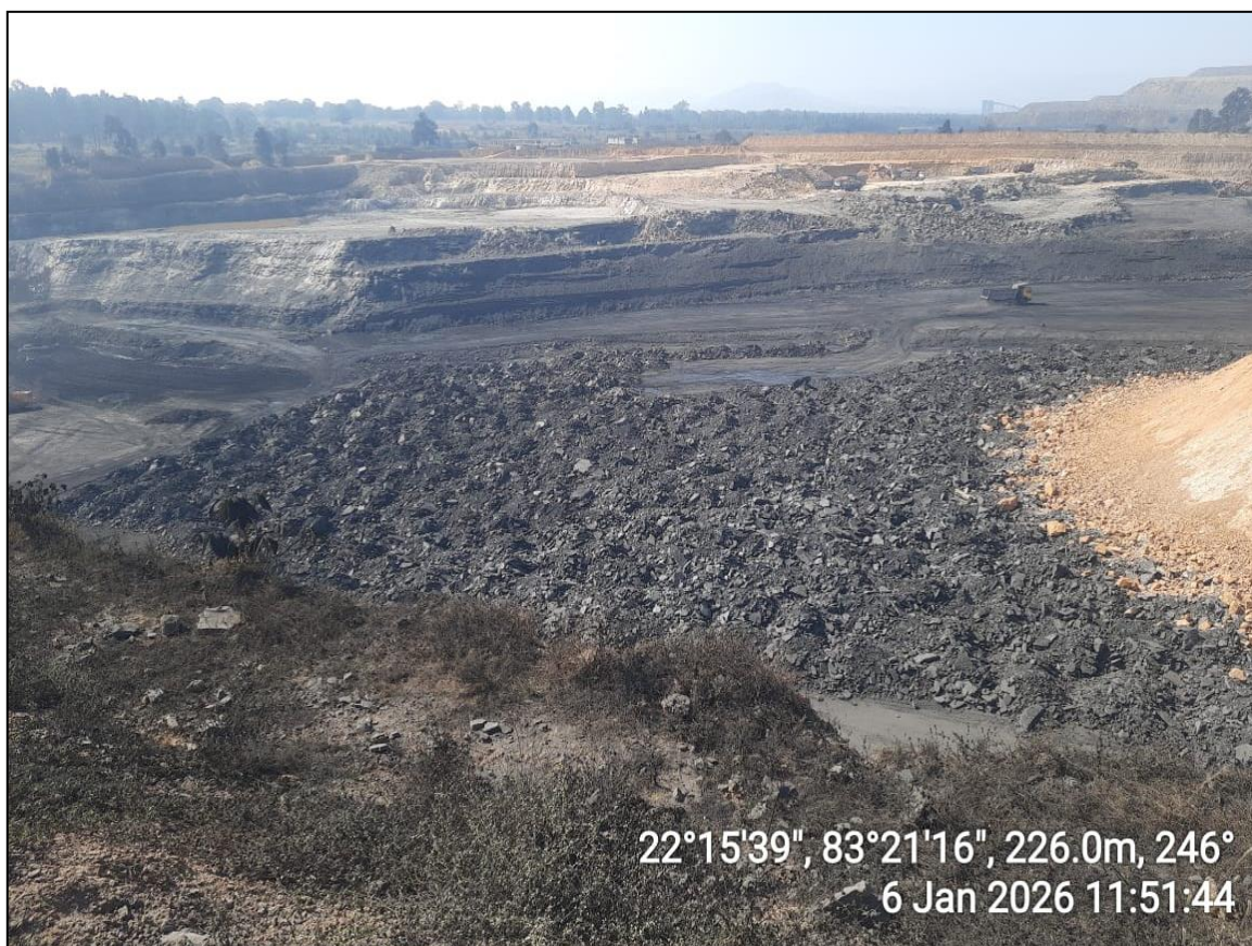
Photo 2.16: Overview of Bijari Opencast Project
