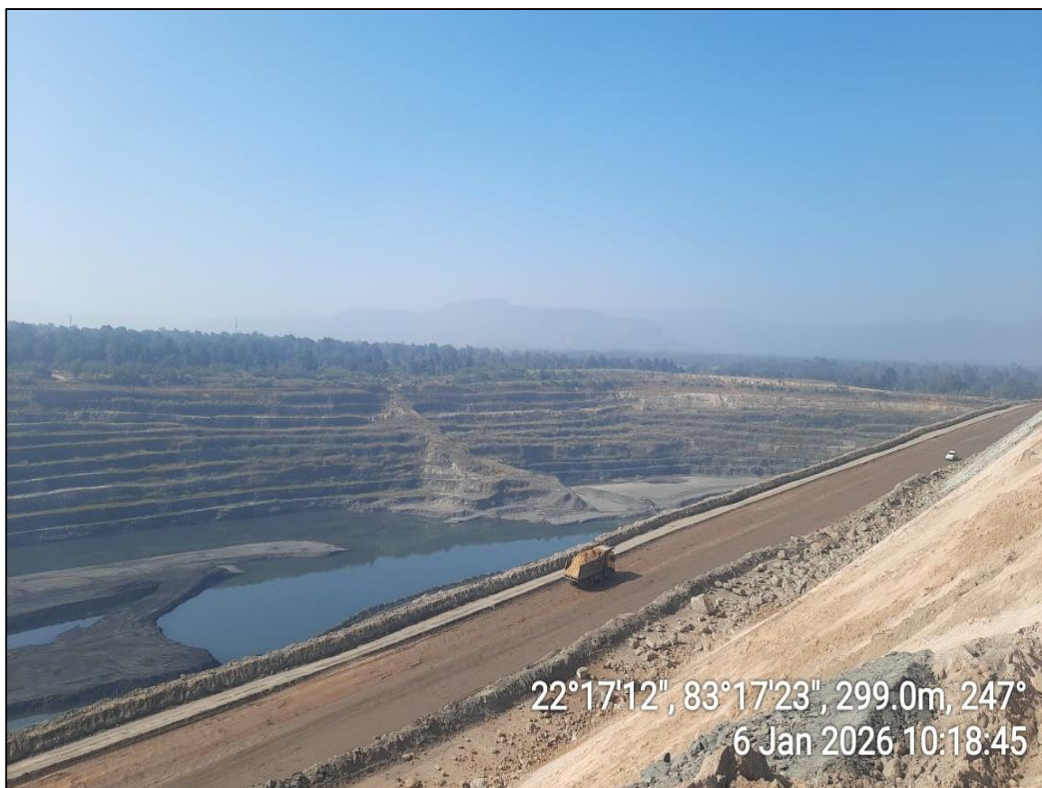
Photo 2.13: Overview of Jampali Opencast Project
