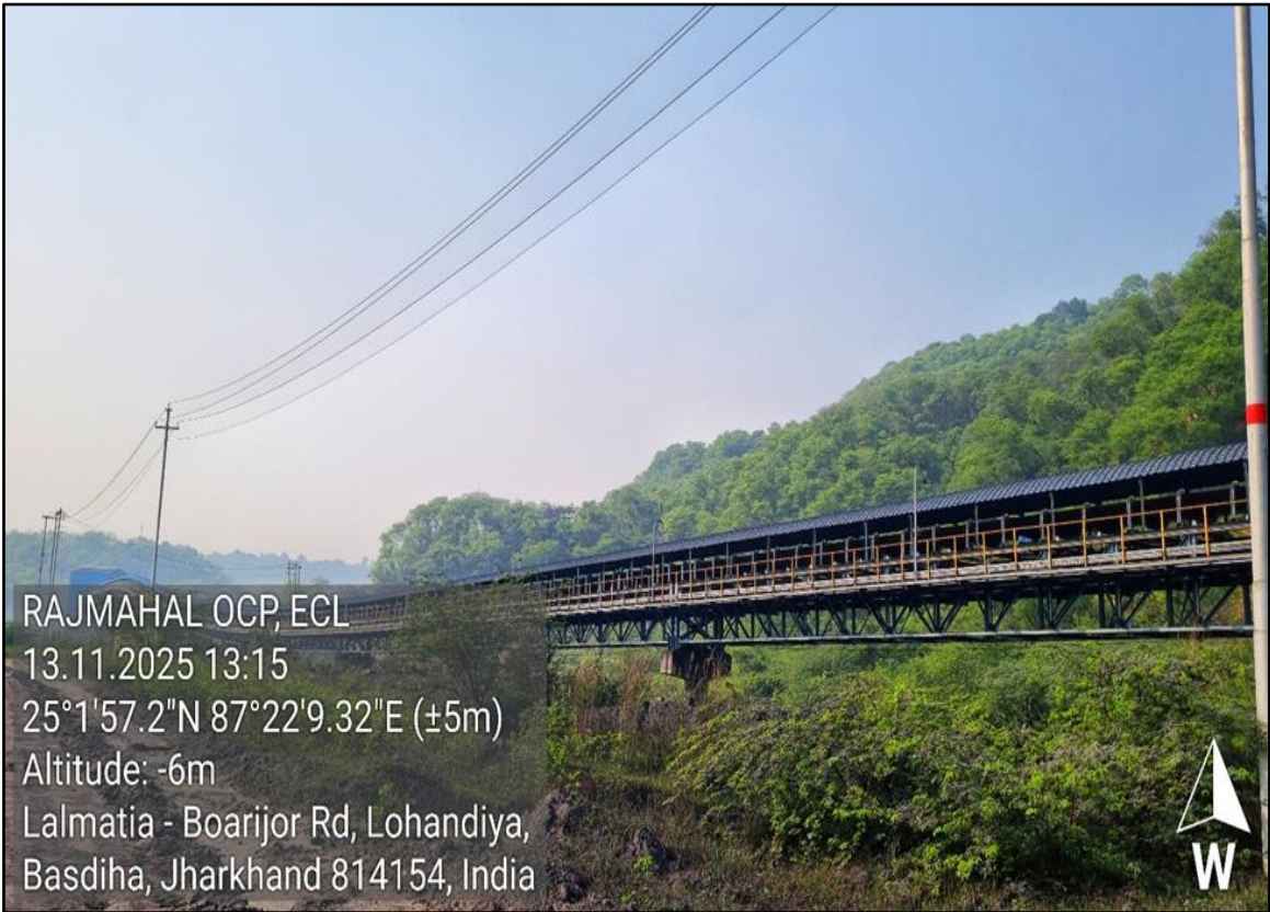
Photo 10.1: Plantation on Backfilled area in Rajmahal OCP, ECL
