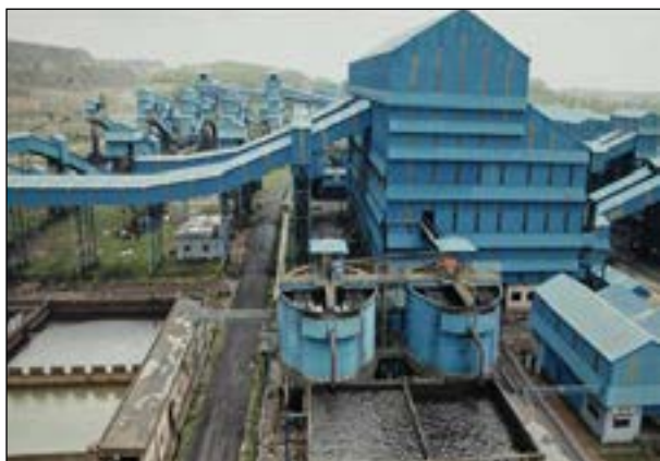
Figure 6 : Washery Plant at IB Valley Lakhampur-MCL (Design Scrutiny)
