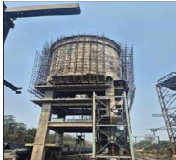
Figure 8: SILO Construction at RG3 OC, Singareni (SCCL)
